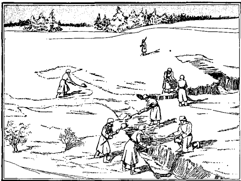
Figure 64.—Camouflaging trenches with willow frames.
